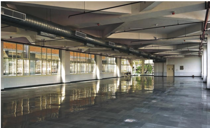
Cross bracing the beams diagonally distributes load while maintaining a thin profile
