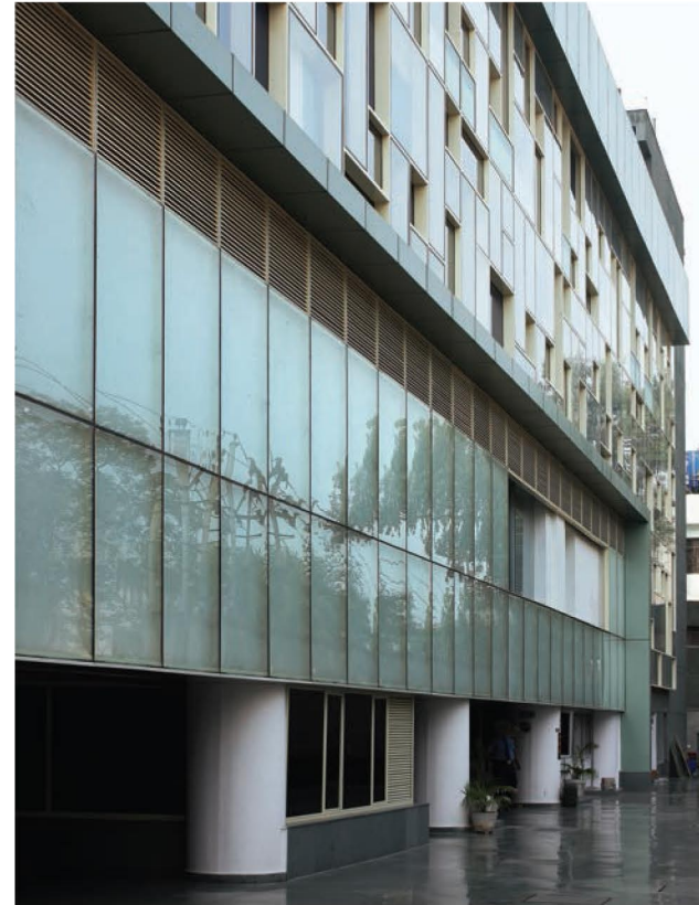
Limiting the columns to the periphery, allows easy expansion to the upper floors and freeing up ground space for vehicular movement
