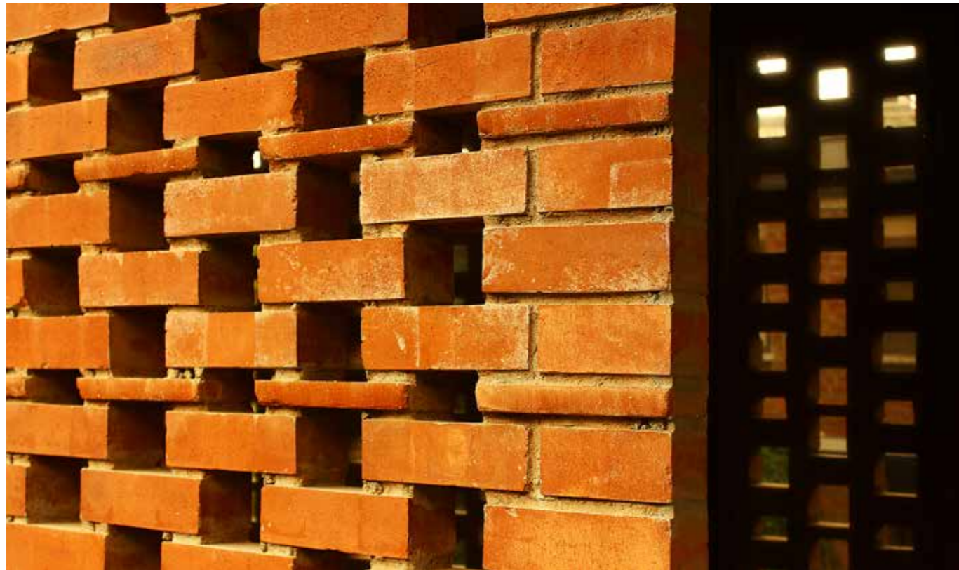
↑ Regular sized and thin bricks combined to create the jalis.
