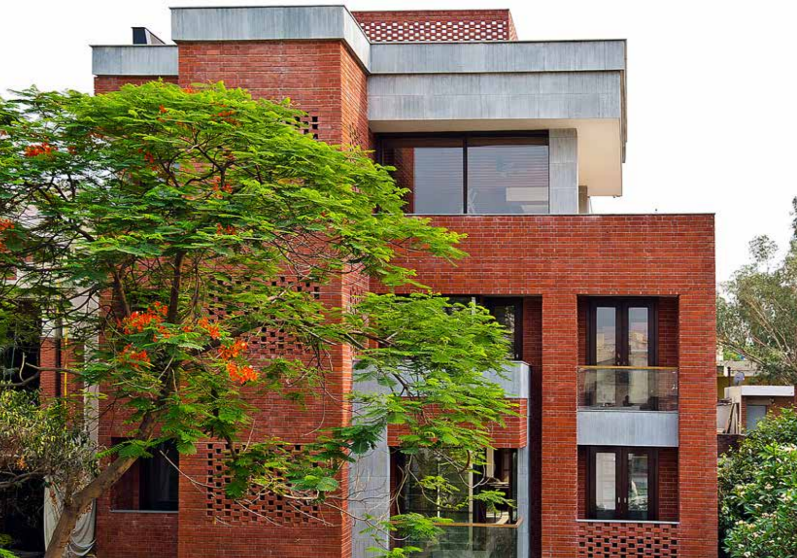
↑ Exterior - Front Façade
