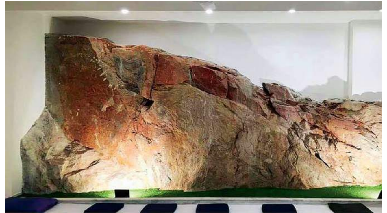
The conversational piece of the building is certainly the existing rock being retained as a wall and also forming part of the building foundation.
